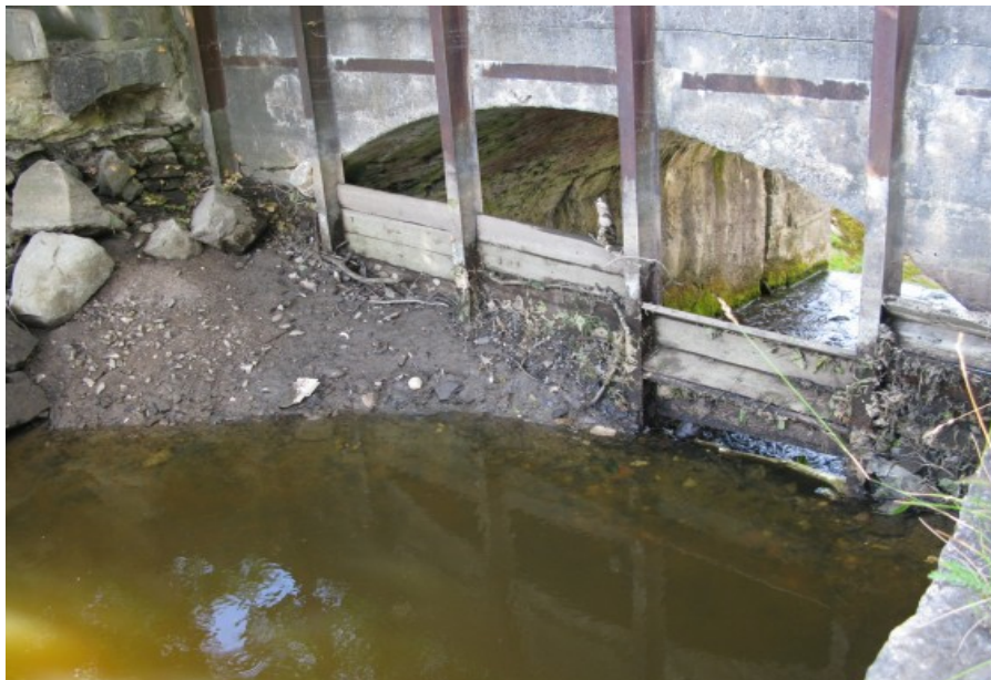
Picture 2 Hydro technical structure with damaged sluice in the Lake Vidusezers, in 2016
